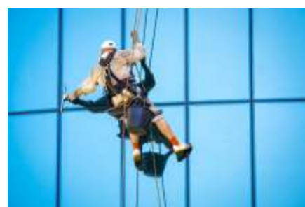
External Cleaning of Glass Facade
